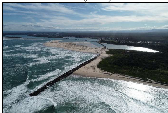
Figure 2 View looking southwest towards Harrington from the ocean, showing the northern breakwater and training wall, and shoaled entrance (27 August 2021)
